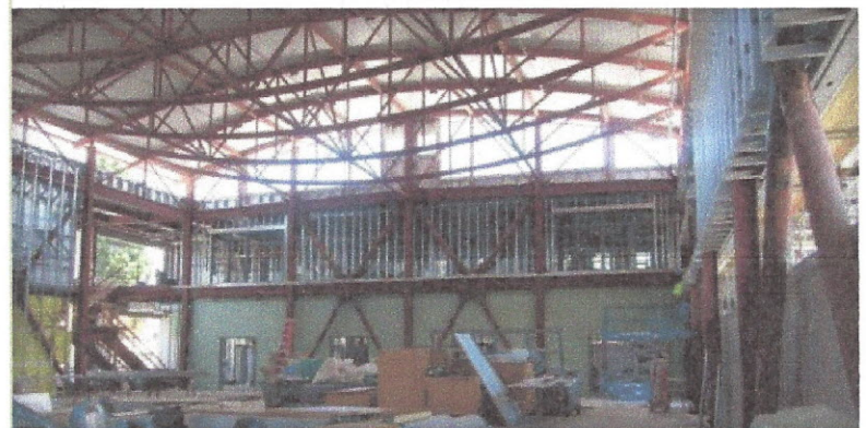
Exterior and interior views of construction at Sylvester Greenwood Academy/LPS.
